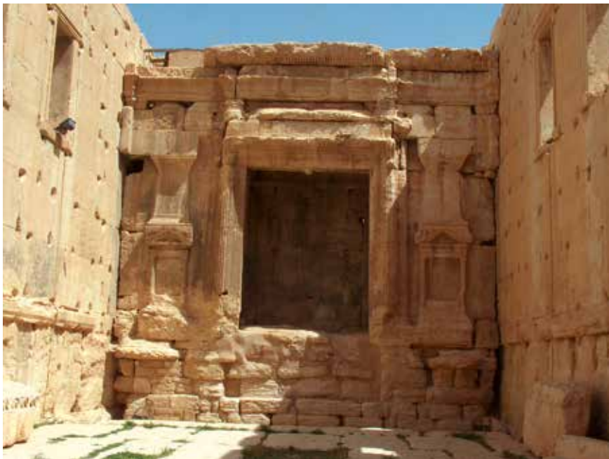
83. The northern adyton inserted between the walls at a short side of the temple. The steps to the niche have not survived
